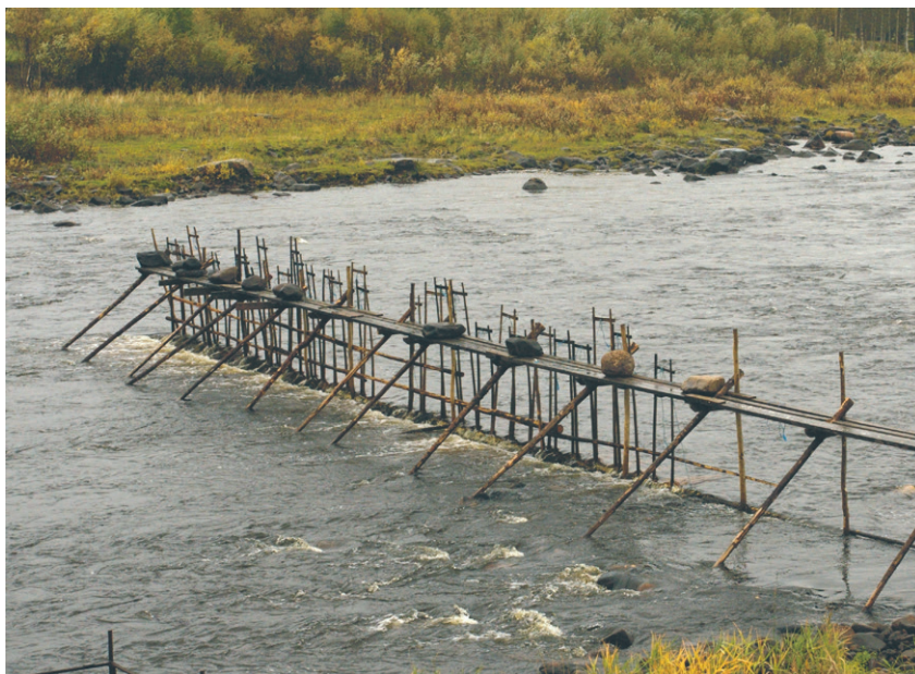
Fig. 50. There is a great variation in construction of the weirs. In the River Simojoki, the weir is constructed of two-legged trestles that are tied together with boards and poles, and with stones to help the construction to withstand the force of the water. 27 September 2011. Photo: Kjell Sjöberg.
