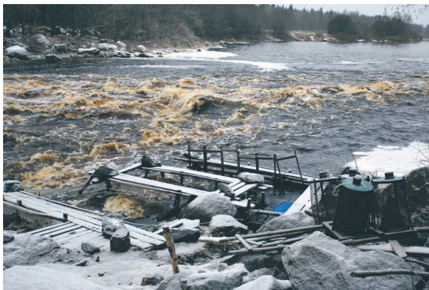
Fig. 55. A weir in River Kyrönjoki with fishing gear formed as a cylinder with a metallic net and the front of plastic net. A wooden tap covers the opening in the trap where the lampreys are emptied. The River Kyrönjoki at Voitby, 29 October 2012. Photo: Kjell Sjöberg.
