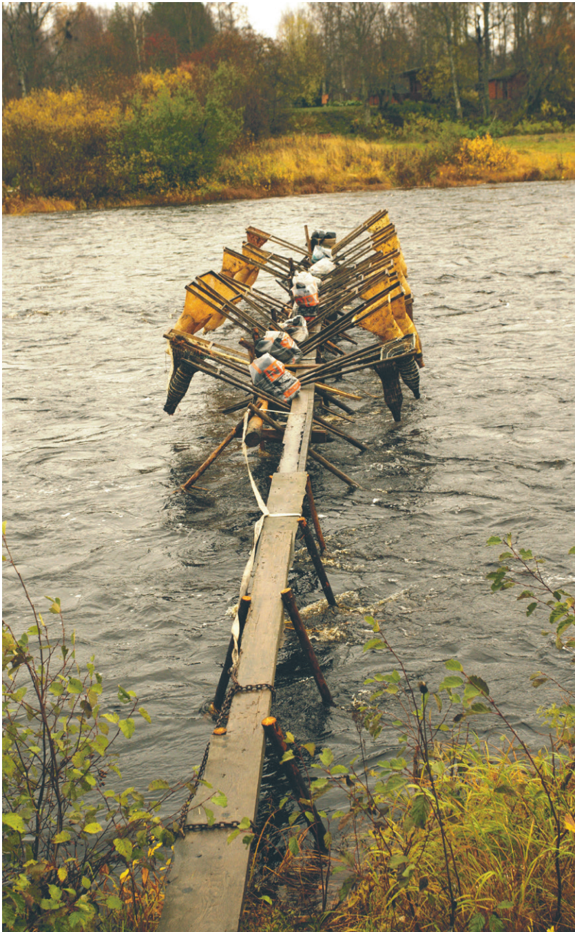
Fig. 52. Another weir of a single row of trestles with traps mostly constructed of glass fibre material. Kuivajoki, 4 October 2012. Photo: Kjell Sjöberg.
