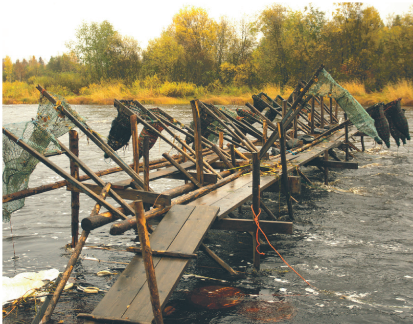
Fig. 53. A more robust weir construction, like here at River Kiiminkijoki, makes it easier for the fishermen to handle the gear. 4 October 2012. Photo: Kjell Sjöberg.
