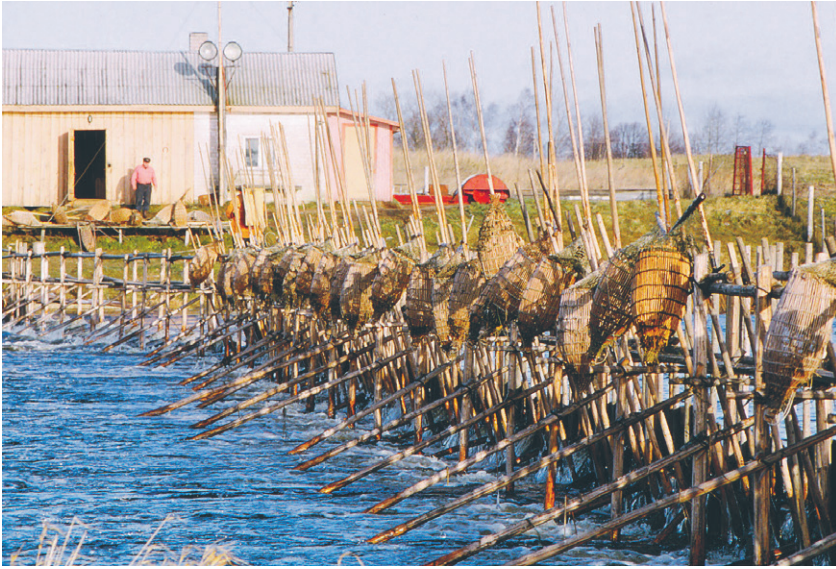
Fig. 65. In weir number 2 from the mouth of the River Salaca, baskets combined with mesh connected to lifting frames were still in use back in 1992. At the building in the background Arnis Rozenšteins is checking the weir. Photo: Kjell Sjöberg.
