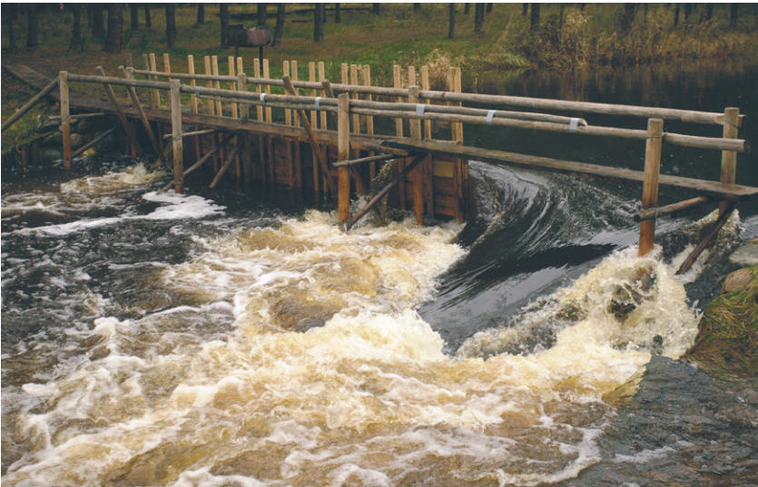
Fig. 82. Weir in the River Svētupe in Eastern Latvia in 2010 where the water stream is partially blocked by a wooden barrier that increases the water level. Gear is placed on this side of the weir with the mouth facing upstream. 16 November 2010. Photo: Kjell Sjöberg.
