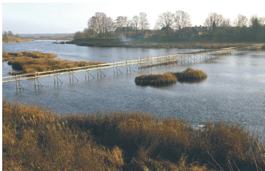
Fig. 94. A difference between Sweden and Finland vs. Latvia is how the gears are placed and constructed. In the River Salaca in Latvia with fairly calm water and a relatively low water level, weirs are used which cover the whole width of the river, and not necessarily near a rapid as is common in Sweden and Finland. 7 November 2011. Photo: Kjell Sjöberg.
