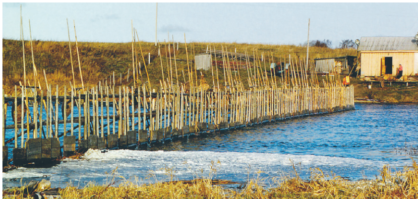
Fig. 78. The same weir as in Fig. 65, but from the other side, where the water is partially stopped by a wooden barrier with openings. The gear are placed on the other side of the weir. The River Salaca in 1992. Photo: Kjell Sjöberg.
