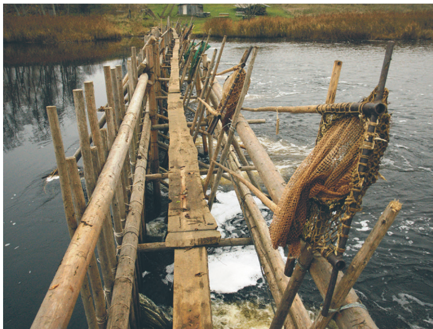
Fig. 71. A close-up of the third weir in the River Salaca with sections of barriers. Note that this barrier has raised the water level at the upstream side to the left. 7 November 2011. Photo: Kjell Sjöberg.
