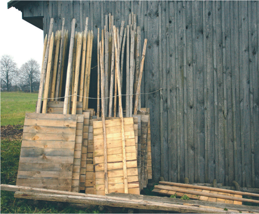
Fig. 81. Details of wooden sections of the type that built up the kind of barrier seen in Figs. 79 and 80. The River Salaca, 7 November 2011. Photo: Kjell Sjöberg.
