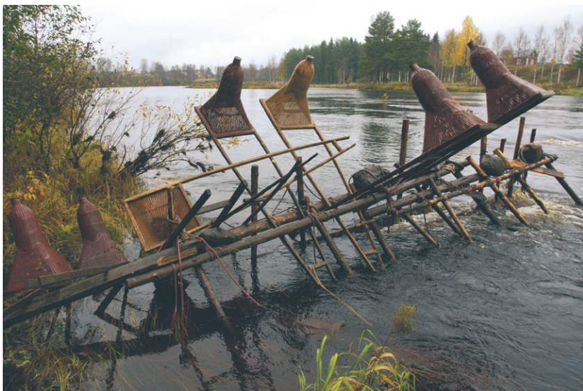
Fig. 51. A weir of a single row of trestles with traps constructed of glass fibre material. Kuivajoki, 4 October 2012. Photo: Kjell Sjöberg.
