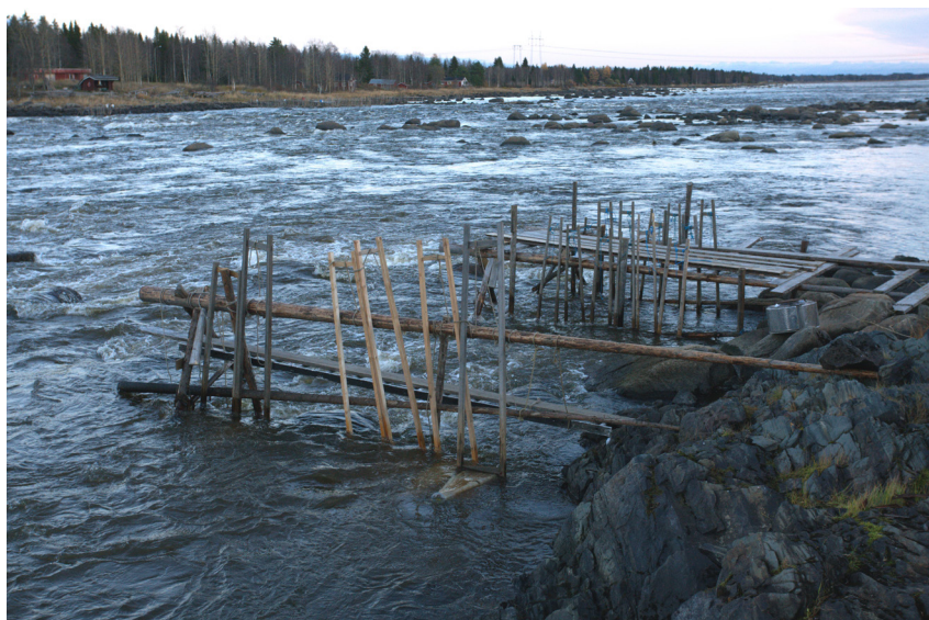
Fig. 24. Lamprey traps attached to two types of weirs, with one and two parallel rows of trestles (Swedish enryggig and tvåryggig strandpata ) in the Rapid Kukkolaforsen on the Swedish side of the River Torneälven/Tornionjoki. 13 October 2010. Photo: Kjell Sjöberg.
