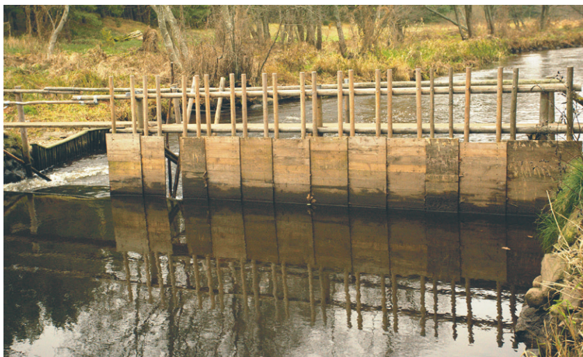
Fig. 83. The same weir as in Fig. 82, but in 2011 with lower water levels. The construction of the wooden barrier can be clearly seen, as well as the opening in the barrier where mesh gear with a lifting frame is placed on the other side of the barrier. 8 November 2011. Photo: Kjell Sjöberg.
