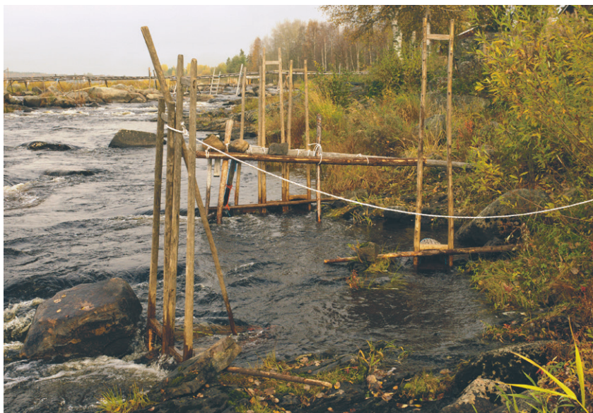
Fig. 57. In the big rivers too, it is possible to find stretches with calmer water flow where the gear could be attached to more simple pata constructions, where the gear is placed just a few together or one by one. The Finnish side of the River Torneälven/Tornionjoki, at the Rapid Kukkolaforseen, 26 September 2011. Photo: Kjell Sjöberg.
